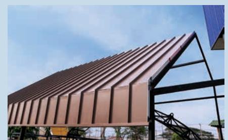
7. Continue fixing next CozyClip and Sandwich Panel until the last panel
