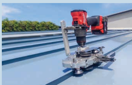
6.2 Seam with Electric Seamer at the edge of each Sandwich Panel
