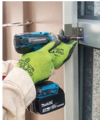
5. Place the second Sandwich Panel and fix third set of CozyClip
