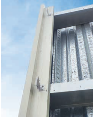
1. Fix the first set of CozyClip in every wall structure
