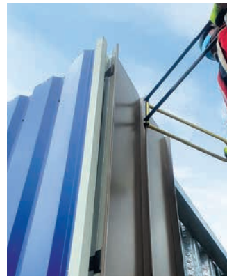
6. Seam with HandSeam and Electric Seamer at the edge of each panel
