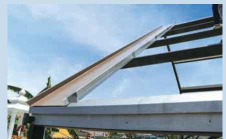
3. Fix the second set of CozyClip in every purlin
