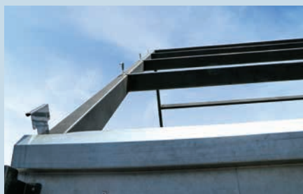
1. Fix the first set of CozyClip in every purlin
