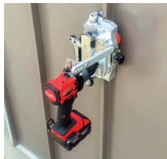
7. Install next Sandwich Panel and CozyClip
