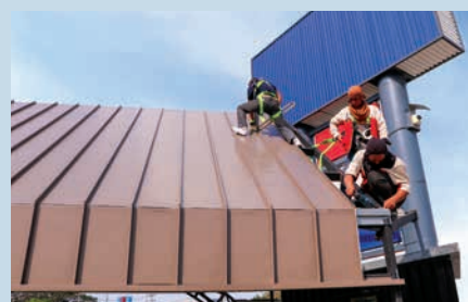
7. Continue fixing next CozyClip and Sandwich Panel until the last panel
