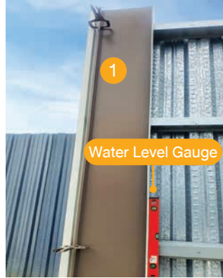
2. Place the first Sandwich Panel over first CozyClip, keep the wall perpendicular by using the Water Level Gauge
