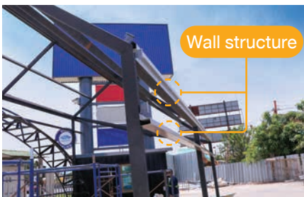
1. Install wall structure
