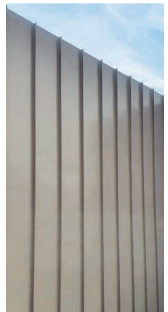
8. Continue fixing next CozyClip and Sandwich Panel until the last panel
