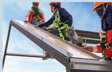
2. Place the first Sandwich Panel over the CozyClip properly
