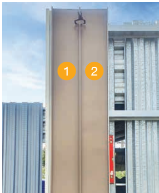
5. Place the second Sandwich Panel and fix third set of CozyClip
