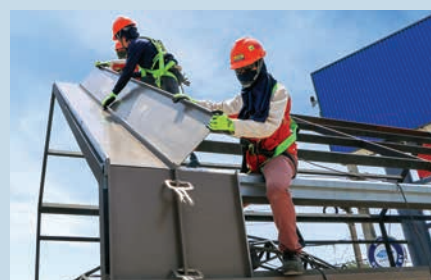
5. Place the second Sandwich Panel and fix the third set of CozyClip
