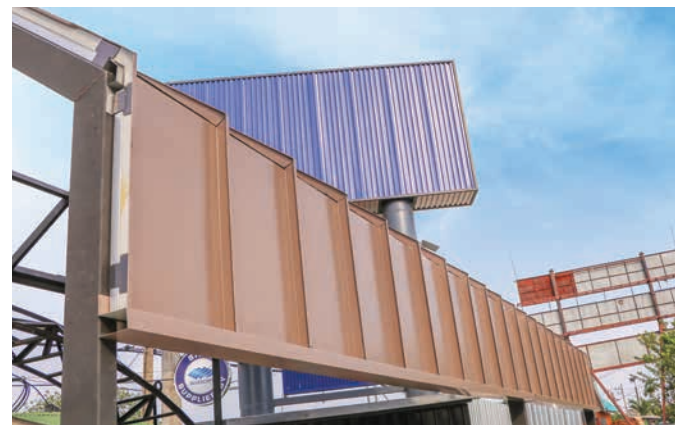
5. After installing the wall panel
