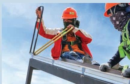
4. Engage the panel and first set of CozyClip by Hand Seam
